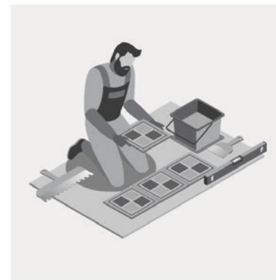
Step-3 Laying of tiles on the Surface
