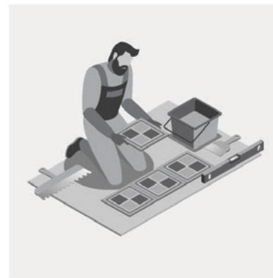
Step-3 Laying of tiles on the Surface
